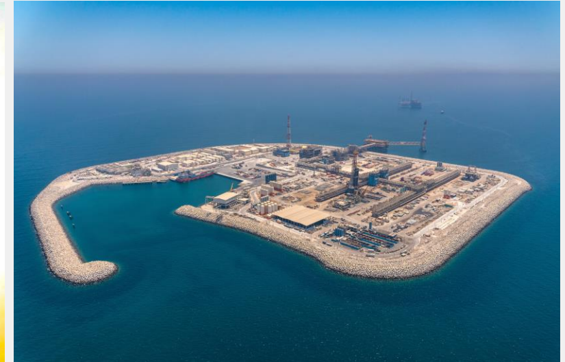
$975 MILLION EPC 2 CONTRACT FOR CONSTRUCTION OF OFFSHORE ARTIFICIAL ISLAND
