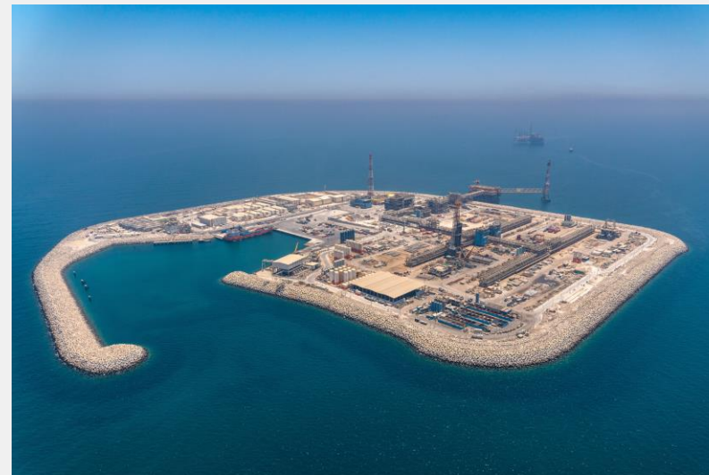
$975 MILLION EPC 2 CONTRACT FOR CONSTRUCTION OF OFFSHORE ARTIFICIAL ISLAND
